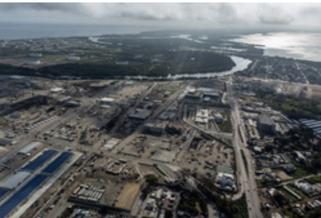
Image: “Pemex Dos Bocas refinery under construction in Tabasco state”, Mexico. Photo: Cesar Rodriguez/Bloomberg https://www.bloomberg.com/news/articles/2022-01-21/mexico-s-crown-jewel-oil-refinery-is-3-6-billion-over-budget?leadSource=uverify%2owall
