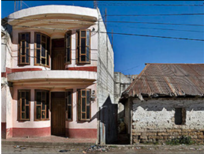
Image: "Remittances architecture" at https://www.bbc.com/mundo/cultura_sociedad/2010/09/100924_galeria_imagenes_mexico_arquitectura_remesas_jp
